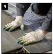
**Install floor finish** Cover the heating cables with self-levelling compound, sand and cement screed or tile directly on top using a full bed of tile adhesive.
