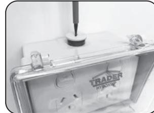
2. Ensure all threaded entries are sealed with silicone sealant or PVC glue. If the rear entries are used ensure the box is sealed well against the wall and that any entries are sealed and water tight to prevent leaks.
