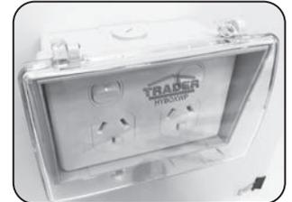
3. Install socket outlet or wall plate accessory and ensure it is securely fastened and that the flap can close fully.
