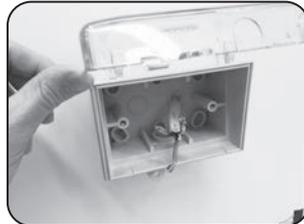
1. When installing the HYBOXWP ensure the product is mounted securely against the wall using the dill points in the covered recesses. Ensure the screw area is well sealed with silicone to protect the IP rating and apply internal screw caps.
