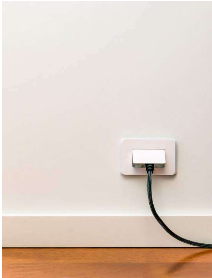
Aesthetically appealing cable management
