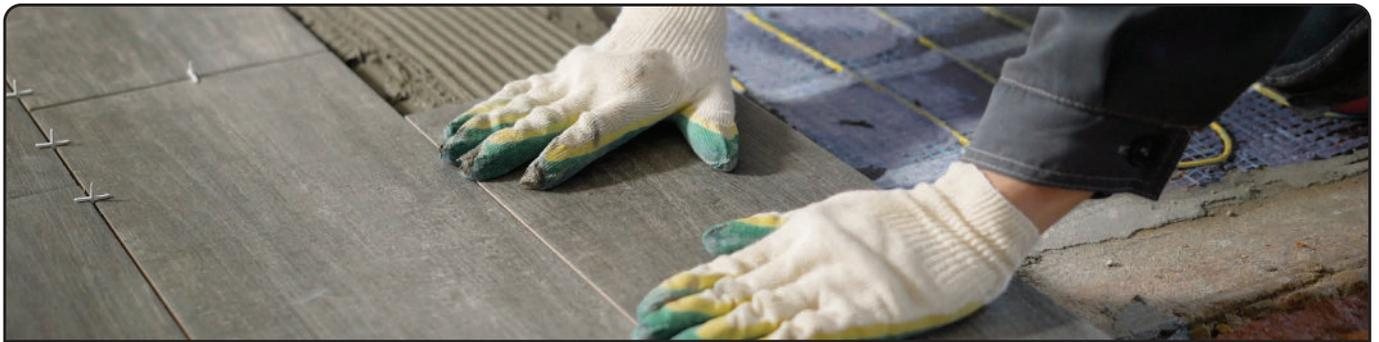
Cover the Thermonet heating with a sand and cement screed or self-levelling compound or tile over using a full bed of tile adhesive. **DO NOT DOT & DAB**
