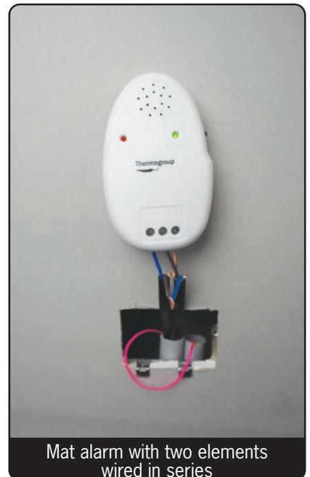
Mat alarm with two elements wired in series
