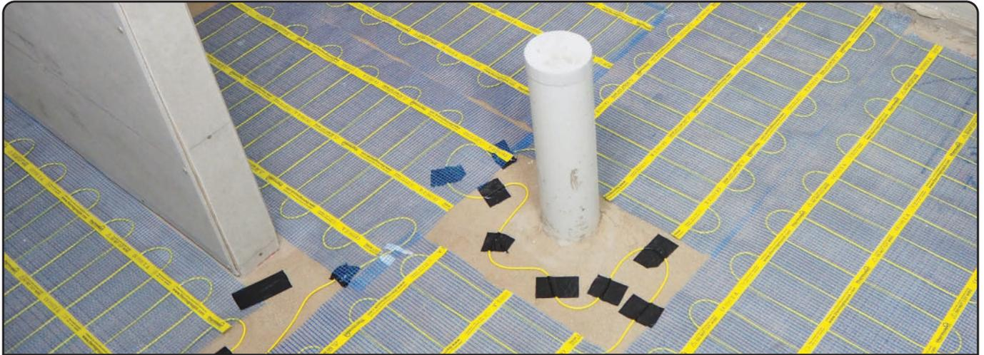
In irregular shaped areas and around fixtures remove the heating cable from the mesh and loose run the cable around the fixture and secure in place with tape.
