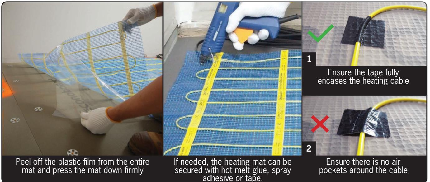
Peel off the plastic film from the entire mat and press the mat down firmly
