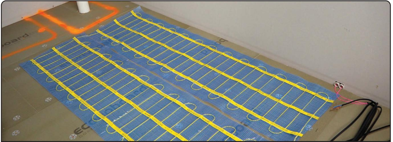
Place the heating mesh in the starting position and roll out the mat until reaching a wall or fixture. Cut the mat (NEVER CUT THE YELLOW HEATING CABLE) and turn the mat 180° and roll it out parallel to the first run.
