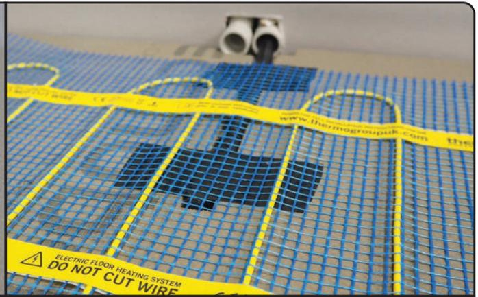
Ensure the floor sensor conduit is located evenly between two runs of heating cable.
